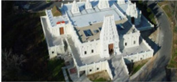
Aerial View of SSVT
